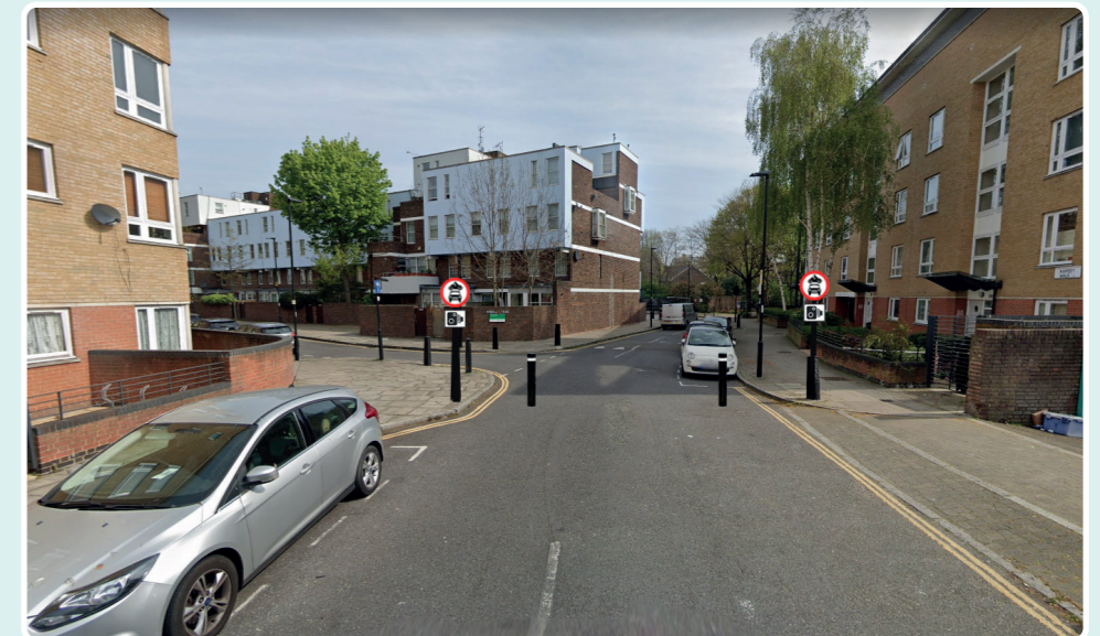
4 Ramsey Walk Camera enforced traffic filter with bollards to narrow roadway, allowing emergency vehicles through. One parking bay suspended.
