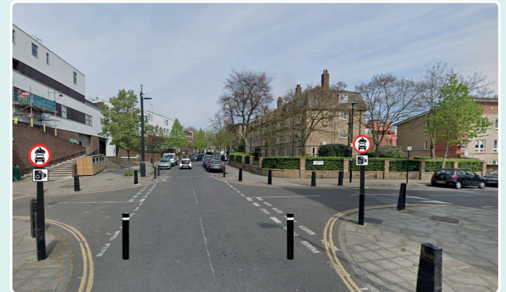
3 Clephane Road Camera enforced traffic filter with bollards to narrow roadway, allowing emergency vehicles through. Two parking bays suspended.
