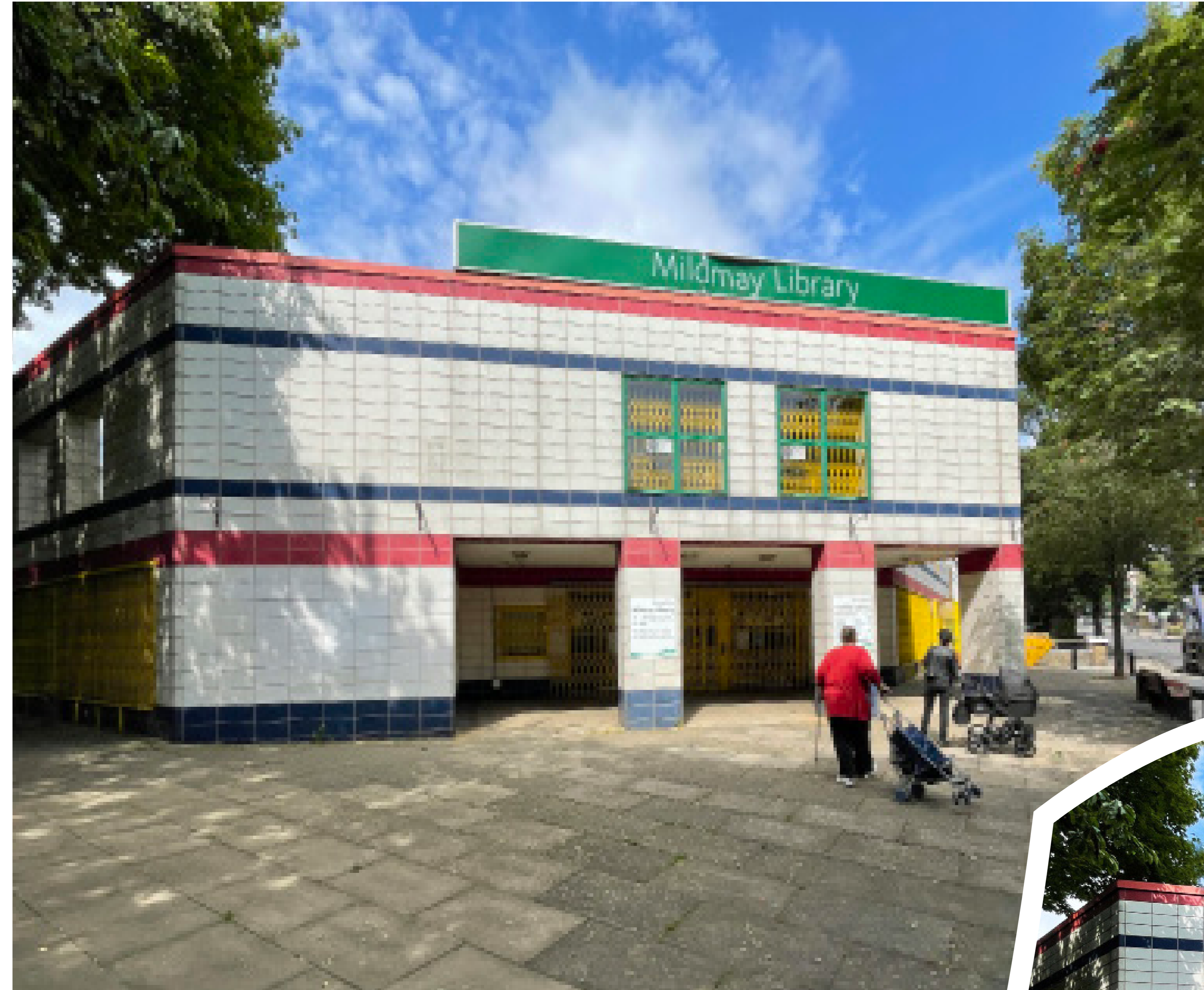
Existing Mildmay Library entrance
