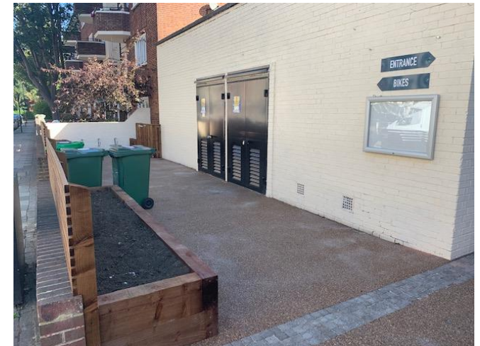
Sebbon St Community Centre improvements
