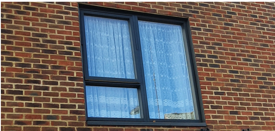
Image 13. Modern double and triple glazed units such as this aluminium composite style can achieve good thermal performance, but they are not appropriate replacements for historic windows/historic style windows because they look so different.
