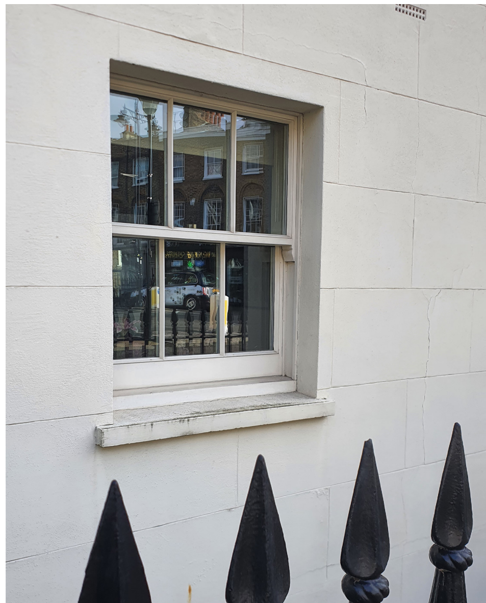
Image 12. Slimline double-glazed window fitted in a replica frame.
