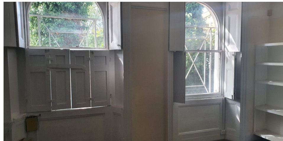
Image 14. Traditional timber shutters with shutter boxes.
