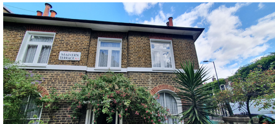
Image 11. The windows in the upper storey have been inappropriately replaced in the past in a way that detracts from the significance of the building. Replacement with slimline double glazing would be appropriate.
