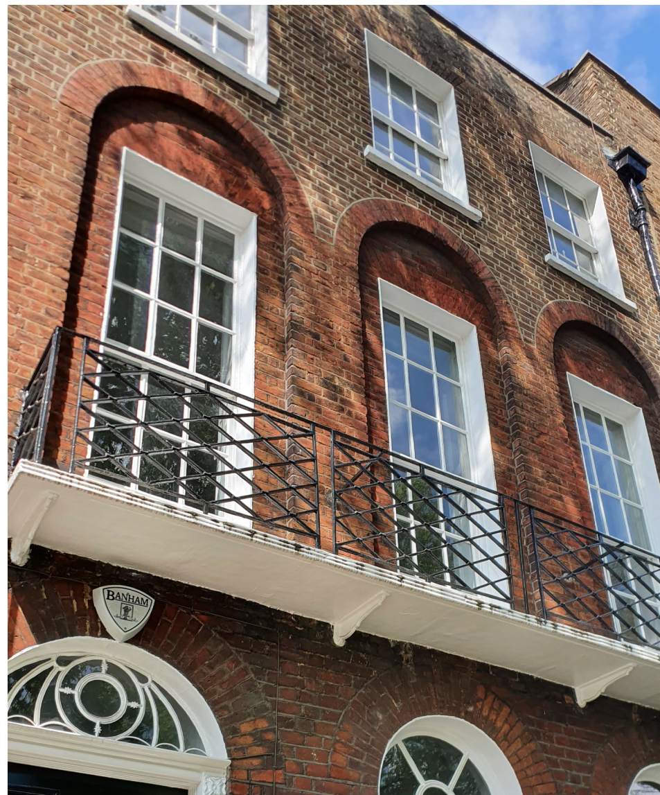
Image 1. Typical windows in a listed building.
