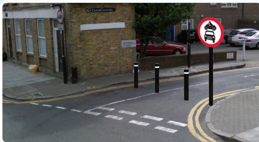
1 Henshall Street Physical traffic filter with bollards
