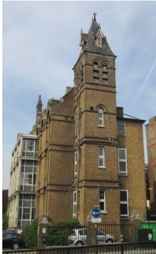
Figure 11 The north wing. Note the extension on the south side (left of picture)
