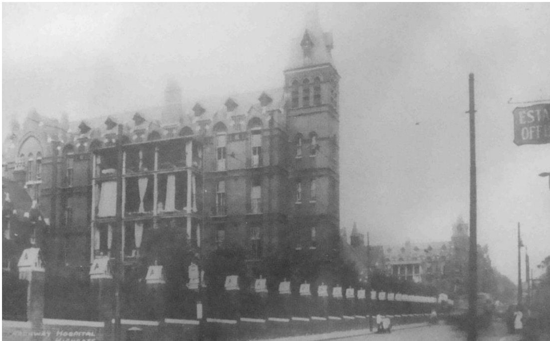
Figure 6 Postcard showing verandas to the north wing of the Holborn Union Infirmary. Note that these were introduced circa 1920s/30s Source: Islington Local History Centre
