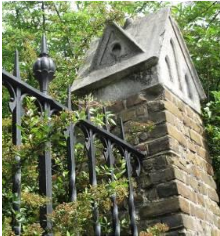
Figure 13 Original railings and piers
