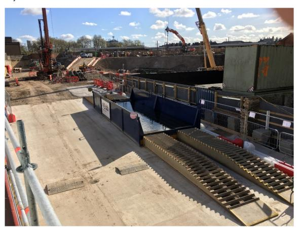
Figure 1: Example of a drive through wheel washing facility
