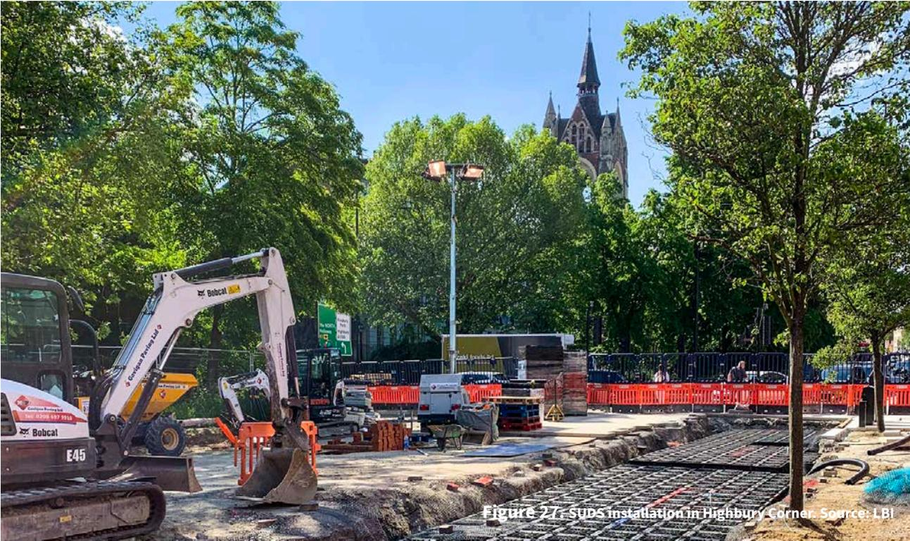
Figure 27. SUDS installation in Highbury Corner. Source: LBI
