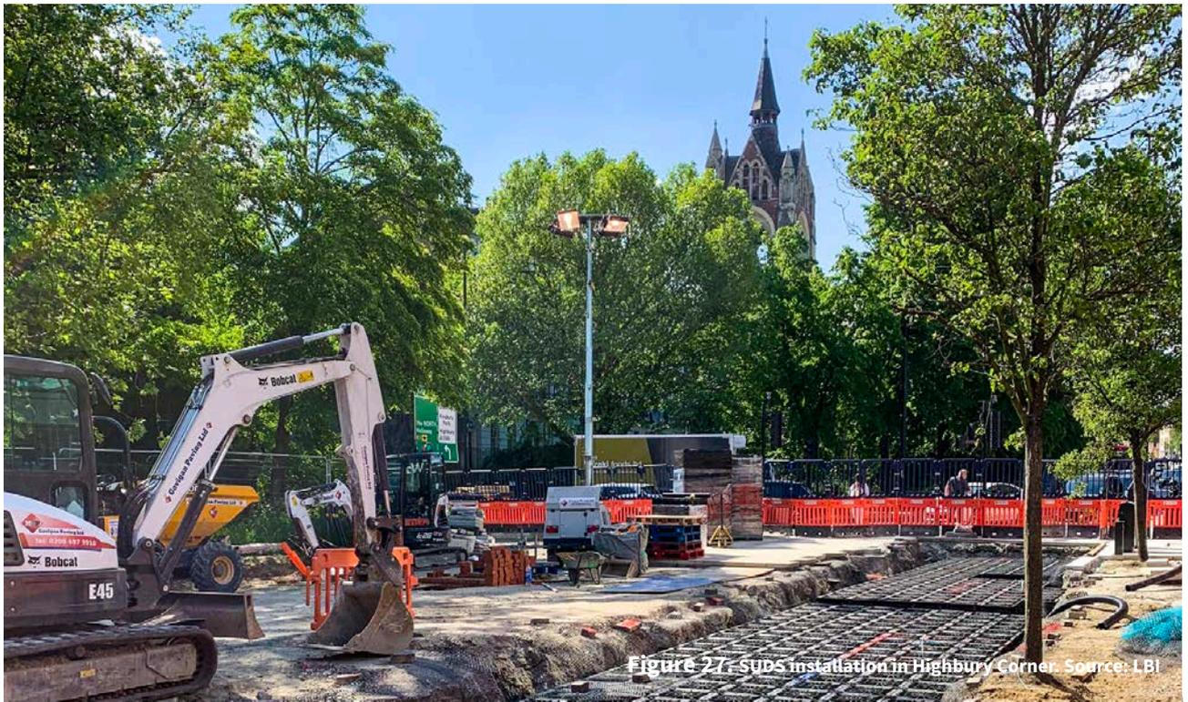
Figure 27. SUDS installation in Highbury Corner. Source: LBI
