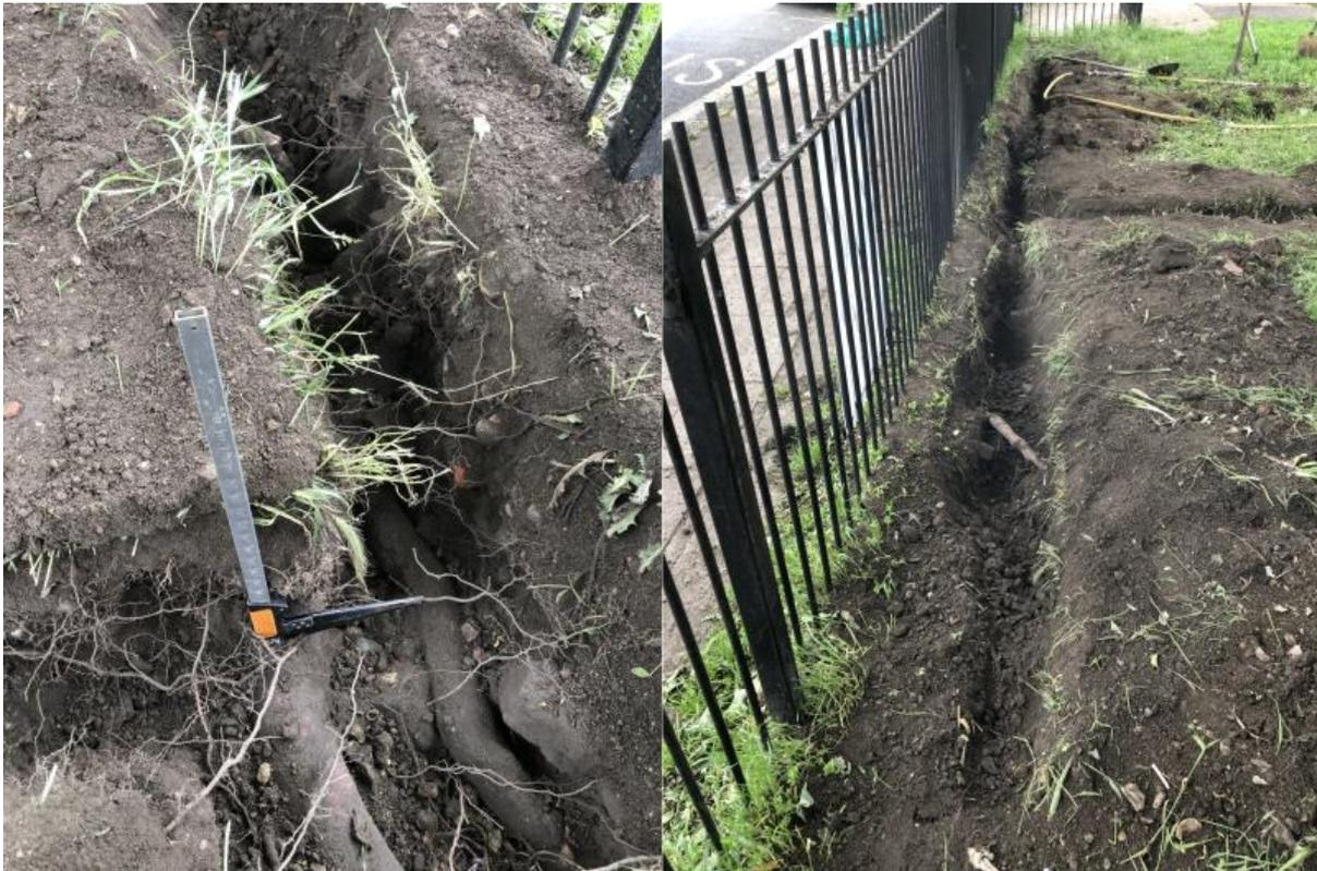
*Photo 10 (left) and Photo 11 (right): Showing roots uncovered from 200mm below ground level from T34, within a trench running parallel with the public footpath to the west.*
