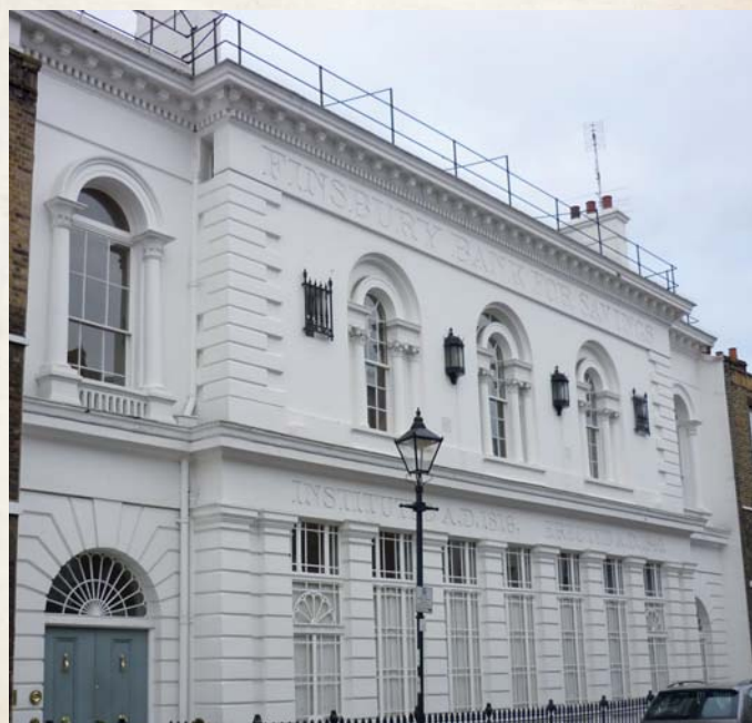
THE FORMER FINSBURY SAVINGS BANK, Sekforde Street, 2010. Dickens deposited funds here in 1845.
