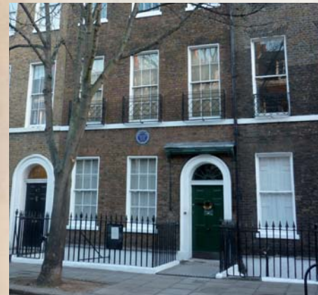
DICKENS HOUSE MUSEUM, 48 Doughty Street, 2011. The building is the only surviving Dickens residence in London.
