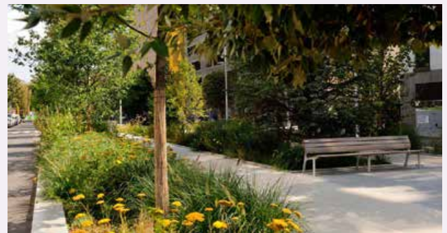
Planting to aid rainwater drainage
