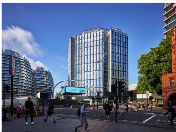
We secured affordable workspace in the highly sought-after White Collar Factory development on Old Street roundabout
