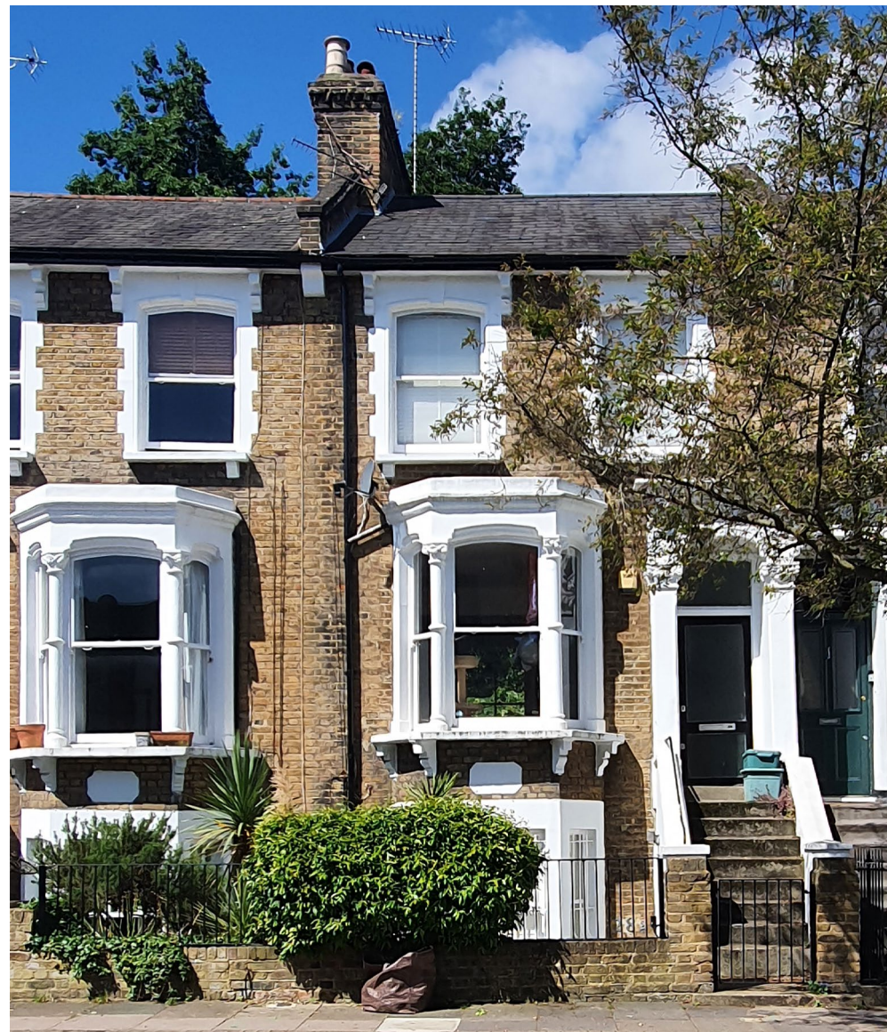
Image 9. Slightly thicker glazed units may be appropriate in windows without glazing bars such as these late 19th century sliding sash windows.
