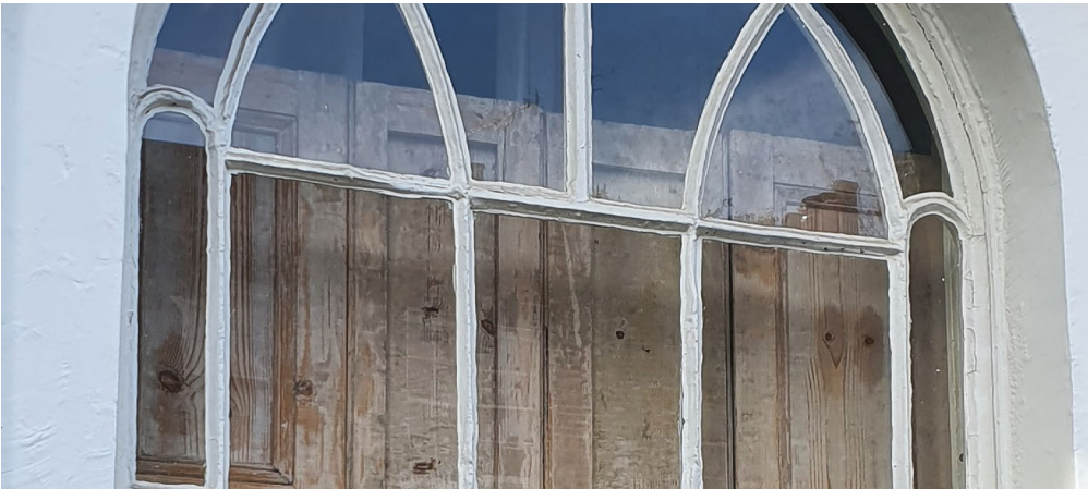
Image 3. Defects to paintwork and putty are common and can be addressed with routine repairs.
