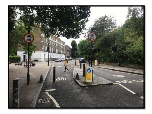
The traffic filter on Colebrooke Row stops through-traffic from using Colebrooke Row as a short cut between Essex Road/Upper Street, New North Road and City Road.
