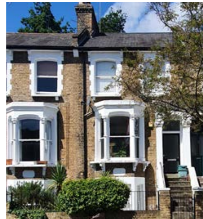
Image 10. Most houses have sliding sash windows without glazing bars at the front.
