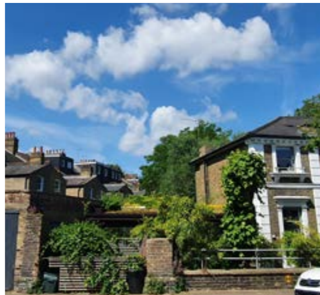
Image 17. Leconfield Road – Green roofs can usually be added to extensions or storage containers
