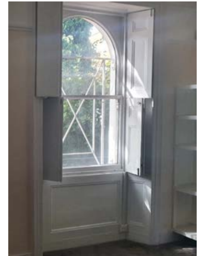
Image 7. Historic shutters can be brought back in to use to reduce heat loss and manage solar gain.
