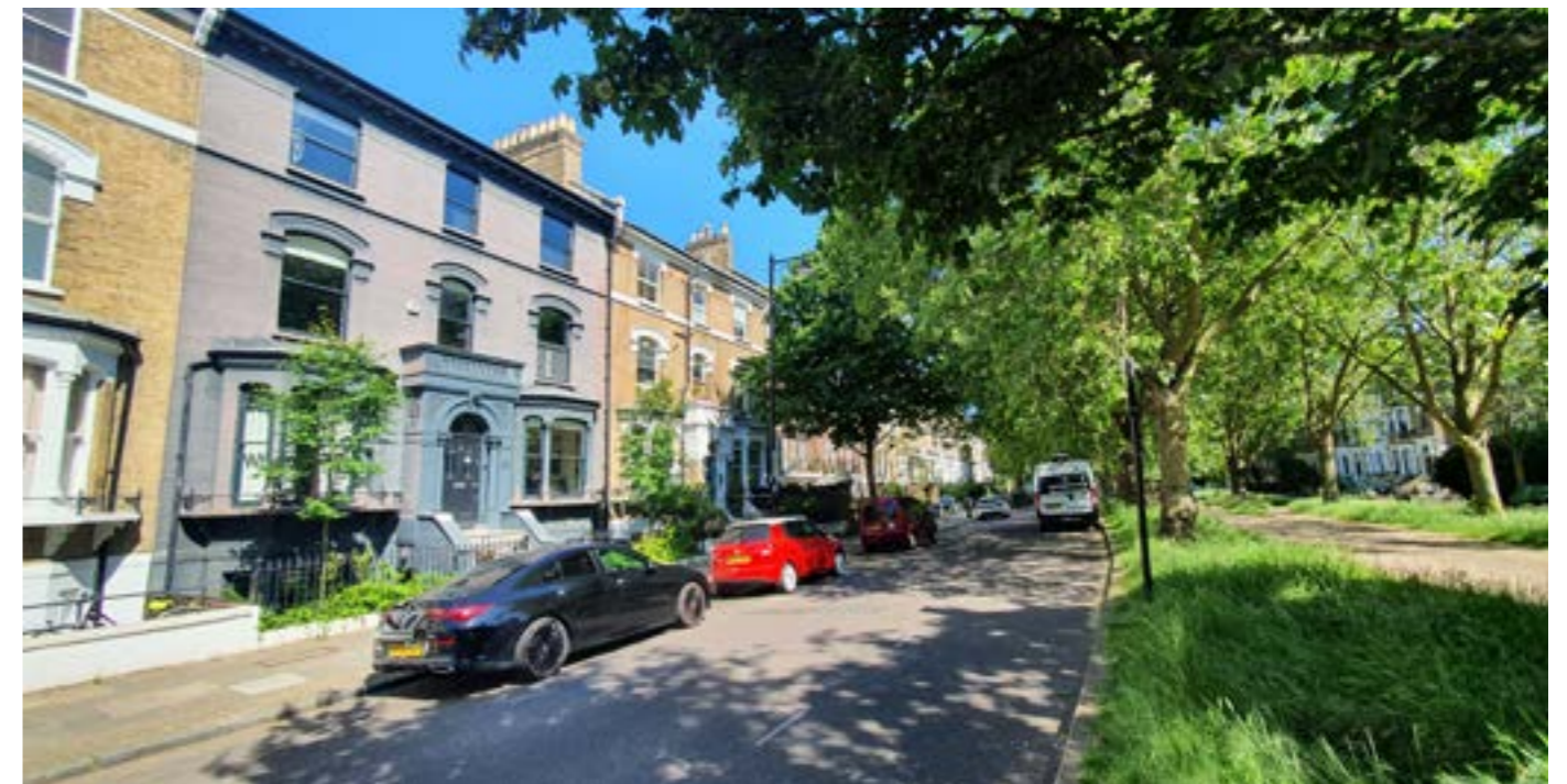
Image 34. Painted brickwork can detract from the appearance of the house and the consistency of the terrace.
