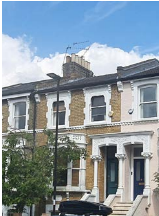
Image 13. Windows on Leconfield Road with evidence of historic blind casings
