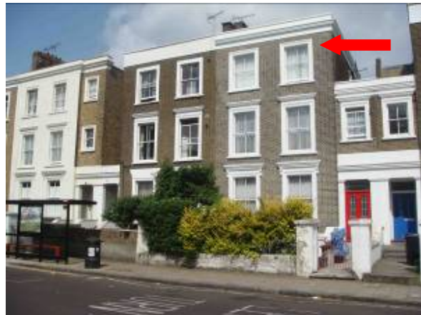
Figure 43 Numbers 48 (right of picture), 50 and 52 (left) Mildmay Park. Note that the principal front elevation to number 52 has been rendered over. The mortar to the brickwork of number 48 has also been poorly applied and finished (arrowed).
