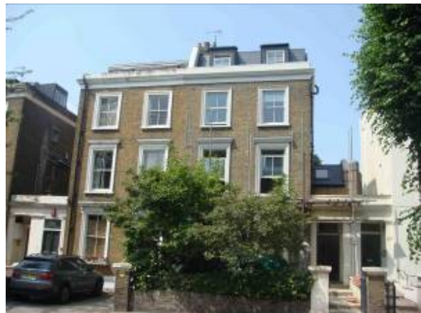
Figure 45 Mansard addition at number 71 Mildmay Park (centre right of picture). Note that this is one of a handful of such additions on Mildmay Park.
