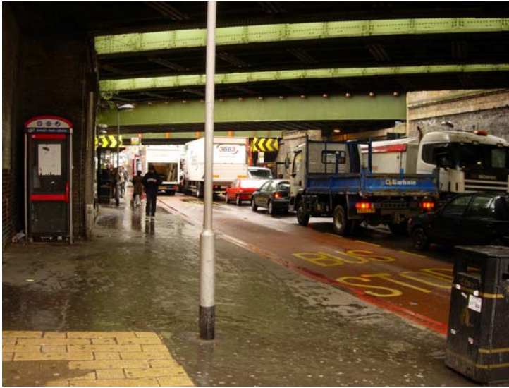
Poor-quality pedestrian environment under Seven Sisters Road railway bridge
