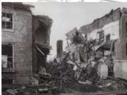
5 Kingsbury Road war damage 1946
