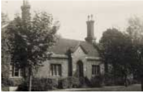
2 Tylers and Bricklayers Almshouses 1830
