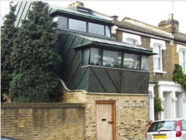
The Venus House projects beyond the established building line of the terrace and has a blank frontage at ground floor level. It was accepted because it replaced an existing structure that occupied the same footprint and because of the exceptional quality of the scheme. Its idiosyncratic character helps give the street local distinctiveness.
