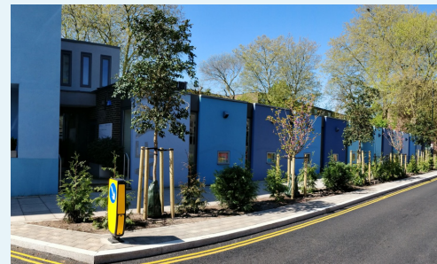
Image: Footway widening and greening
