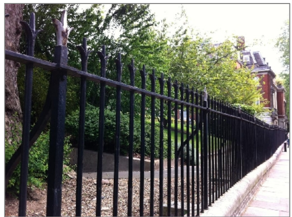
Photo 10: View of perimeter railings on Hardwick Street
