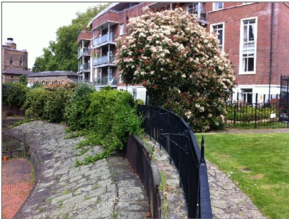
Photo 7: View of Inner Pond revetment with the Nautilus Building, the Engine/Pump House and South Stores behind
