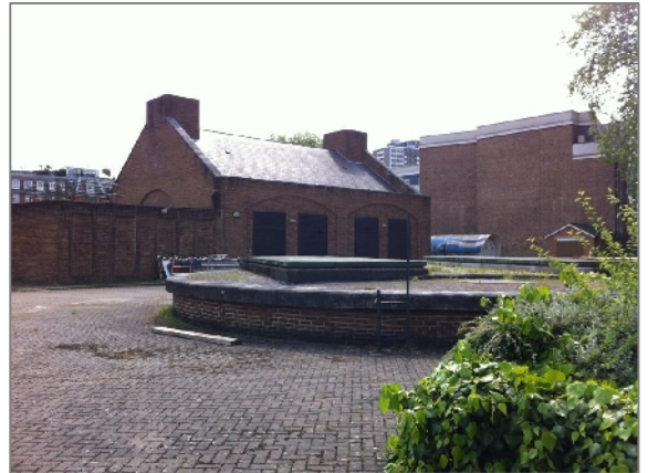
Photo 14: View of Thames Water Ring Main Compound, with Thames Water Pumps and Engine House behind
