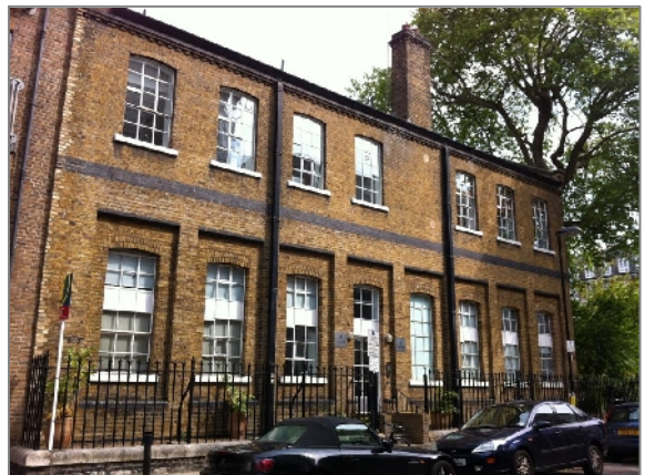
Photo 8: View of Remus Building, looking north
