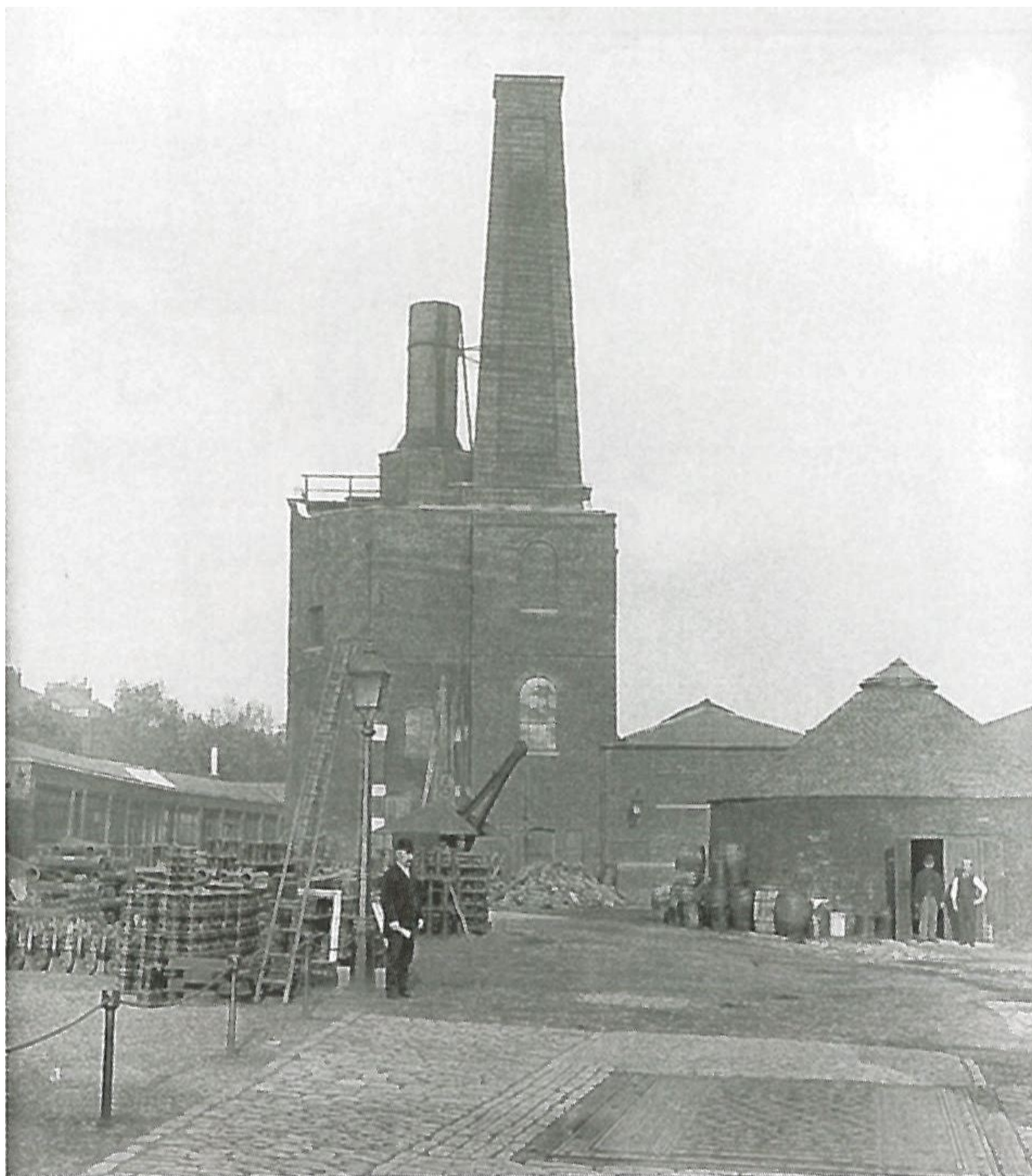
New River Head engine house, early 1900s. London Metropolitan Archives (LMA) photograph
