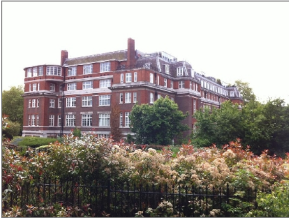
Photo 5: View of New River Head (Headquarters) building, looking south-east
