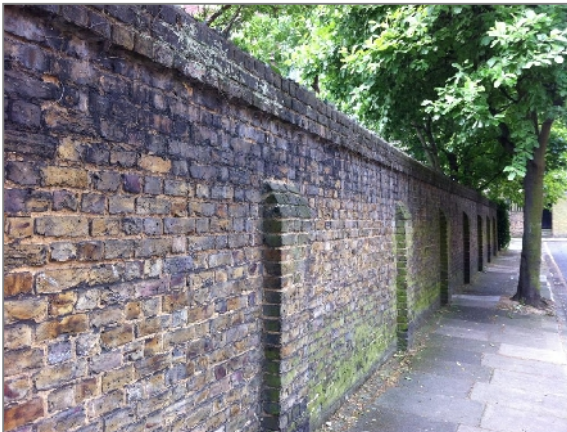
Photo 9: View of brick boundary wall on Myddelton Passage
