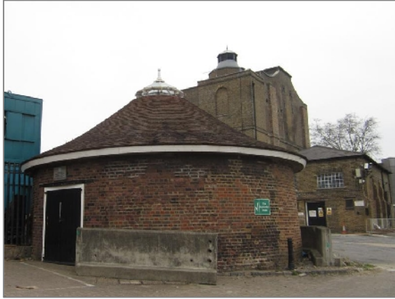
Photo 3: View of Mill Base, looking north-east, with the Engine/Pump House behind,
