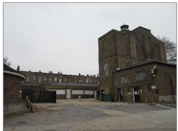
Photo 2: View of the Engine and Pump House, looking north, with the North Stores behind
