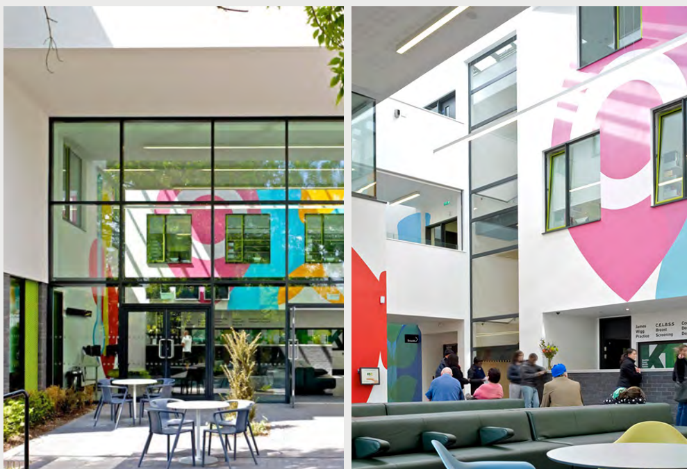
Kentish Town Health Centre - example of new medical services
