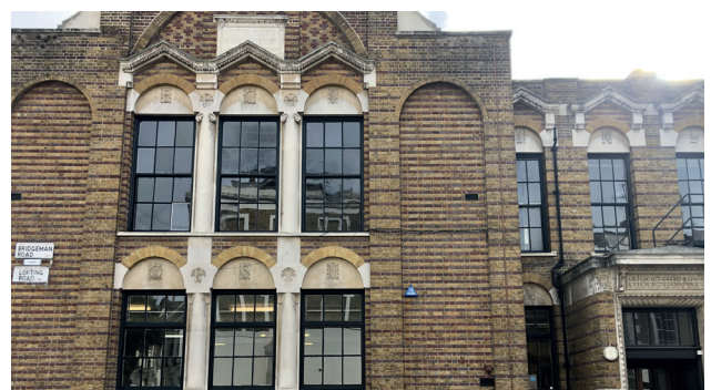
Exterior facade and entrance of West Library
